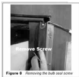
Figure 8 Removing the bulb seal screw
