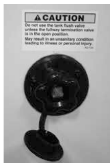
Tank Flush Inlet
