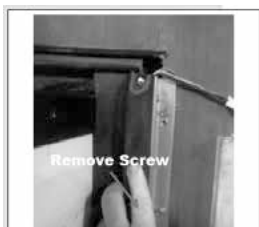
Figure 8 Removing the bulb seal screw
