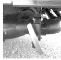
Grey Tank Drain
