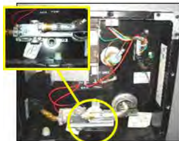
Fig 1: Water Heater Drain Plug
